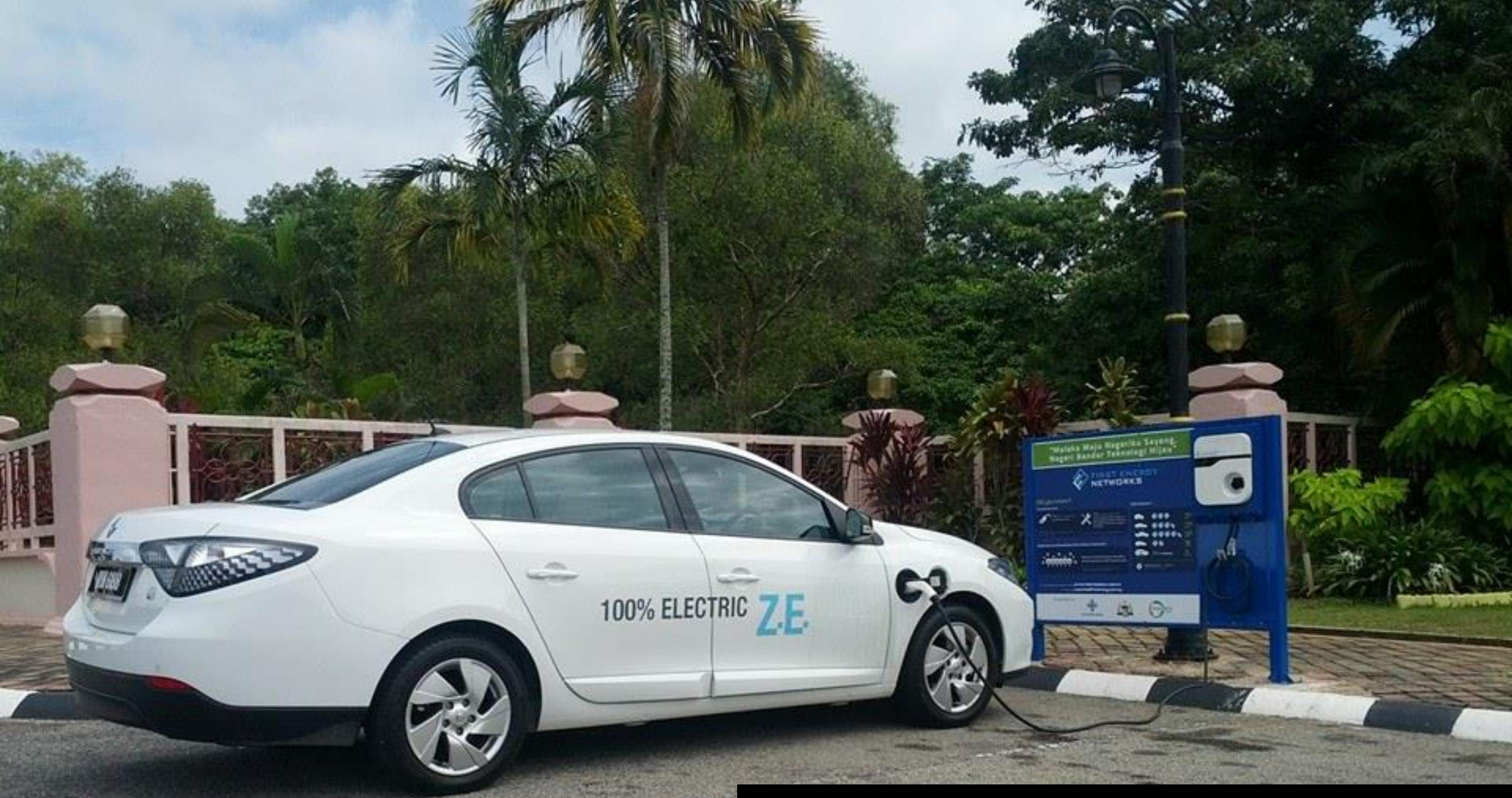
Electric Car Charging Station in Melaka
