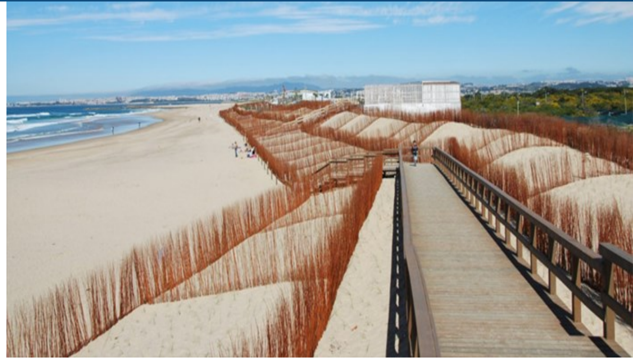
Construction of elevated wooden pathway alongshore and cross-shore
