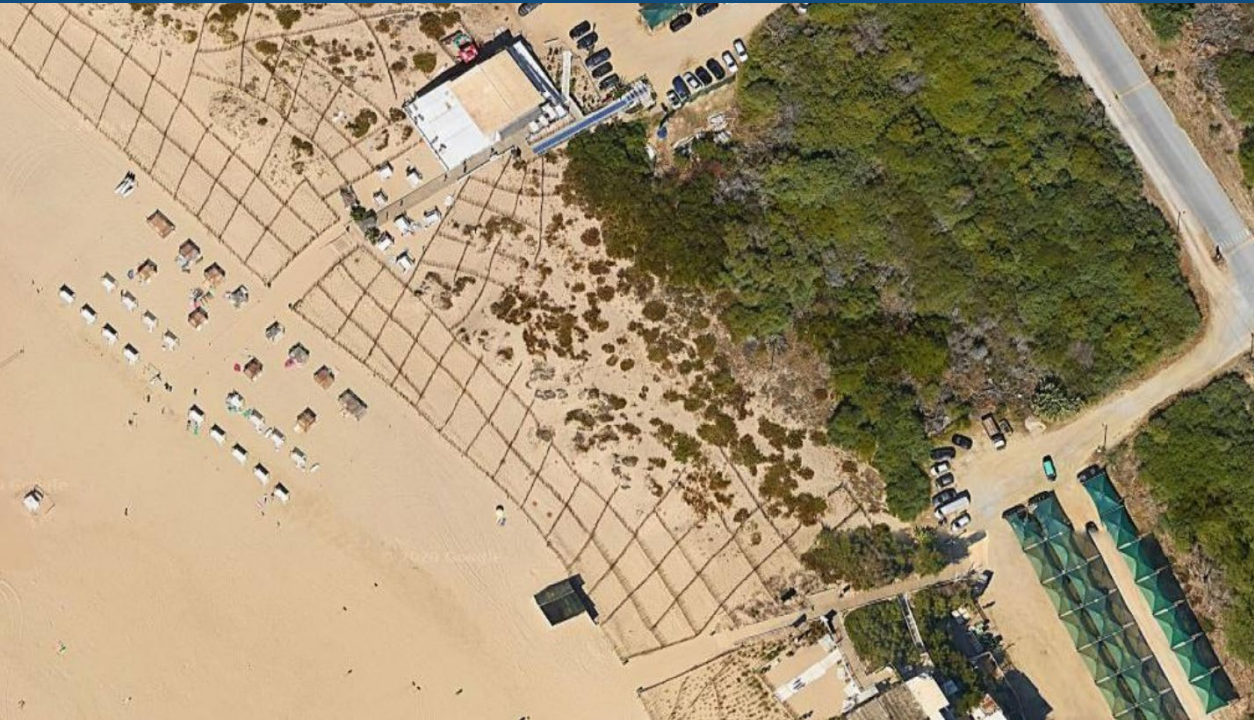
Construction of reticulate fences
